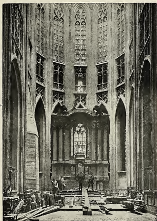
Louvain. Church of St. Peter Interior of the choir after the fire
